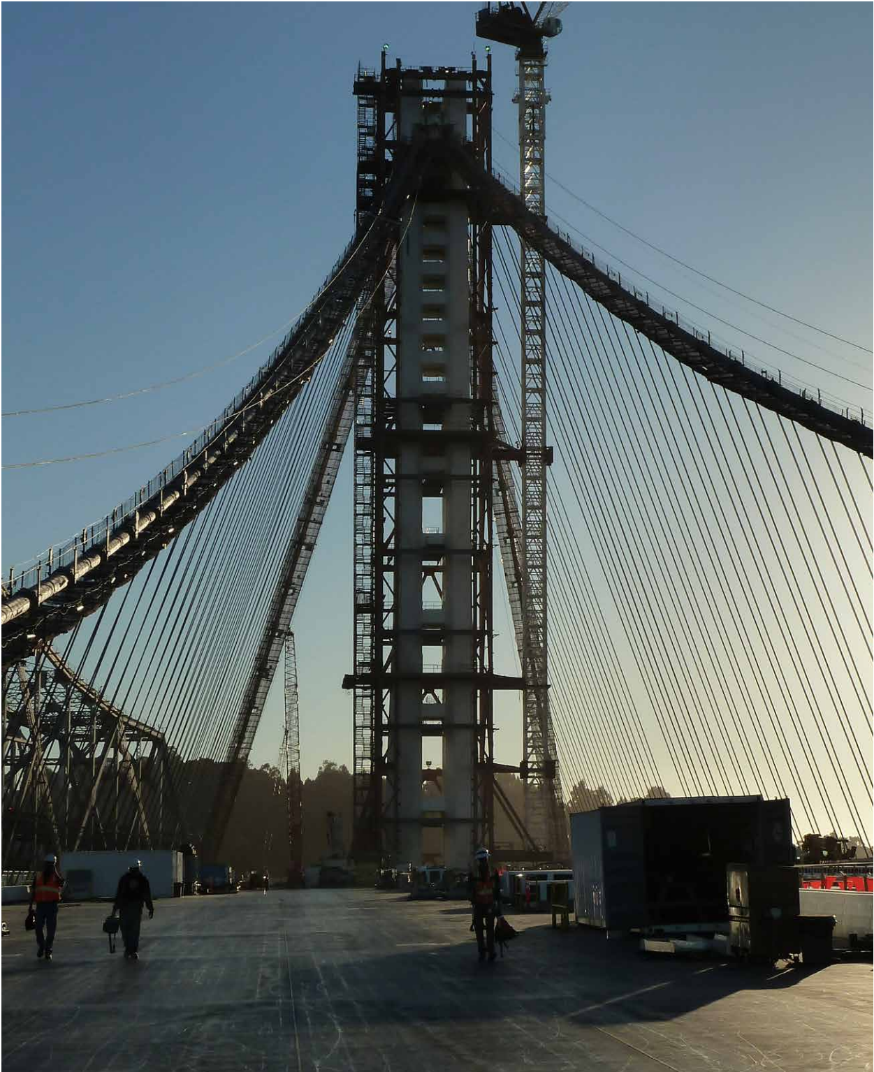
Surface protection work on a steel bridge
