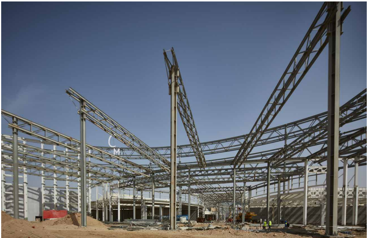
Steel construction and application of passive fire protection in Dubai
