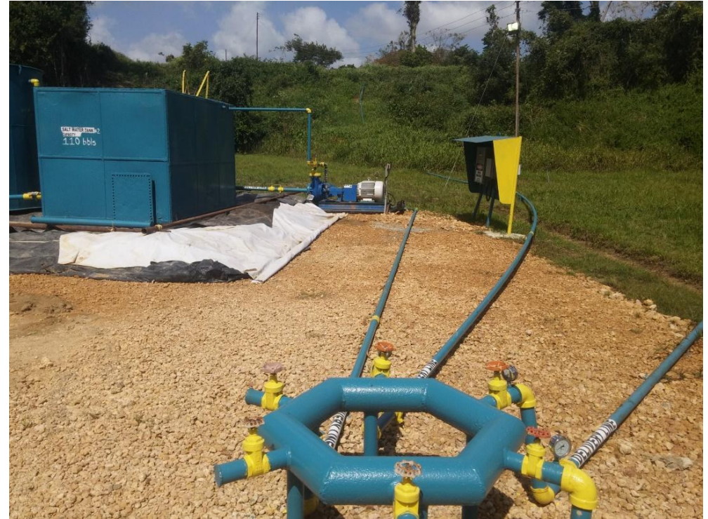
Pipeline network at Morne Diablo field
