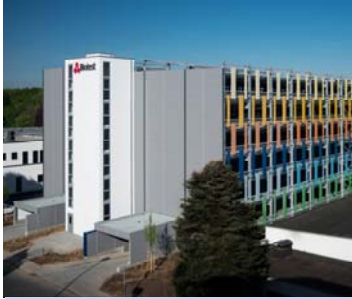
Completed multi-storey car park
